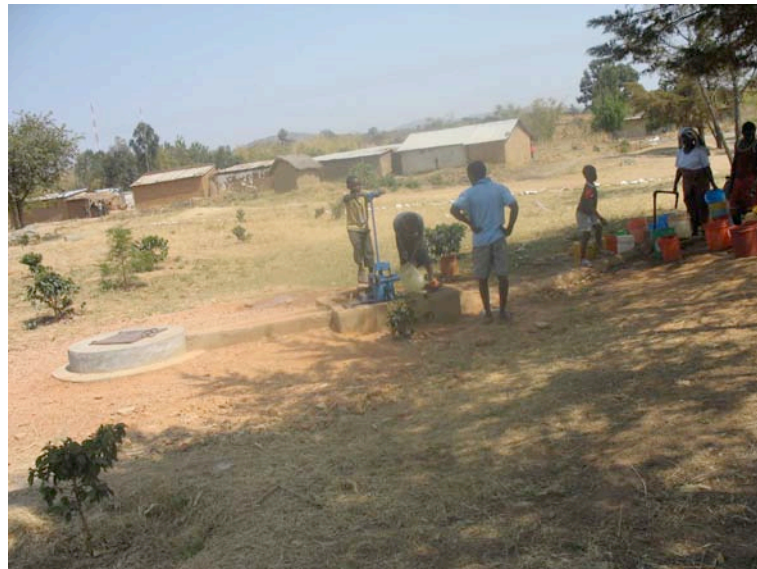
Clean water in Lundamatwe! The borehole is on the left, a child is pumping in the middle and the output is on the right.
