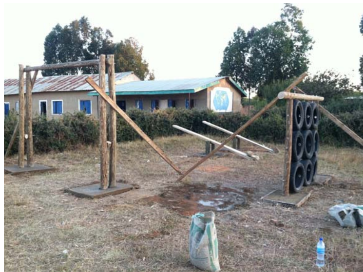
Playground equipment under construction at the Lundamatwe Primary School (July 2012).
