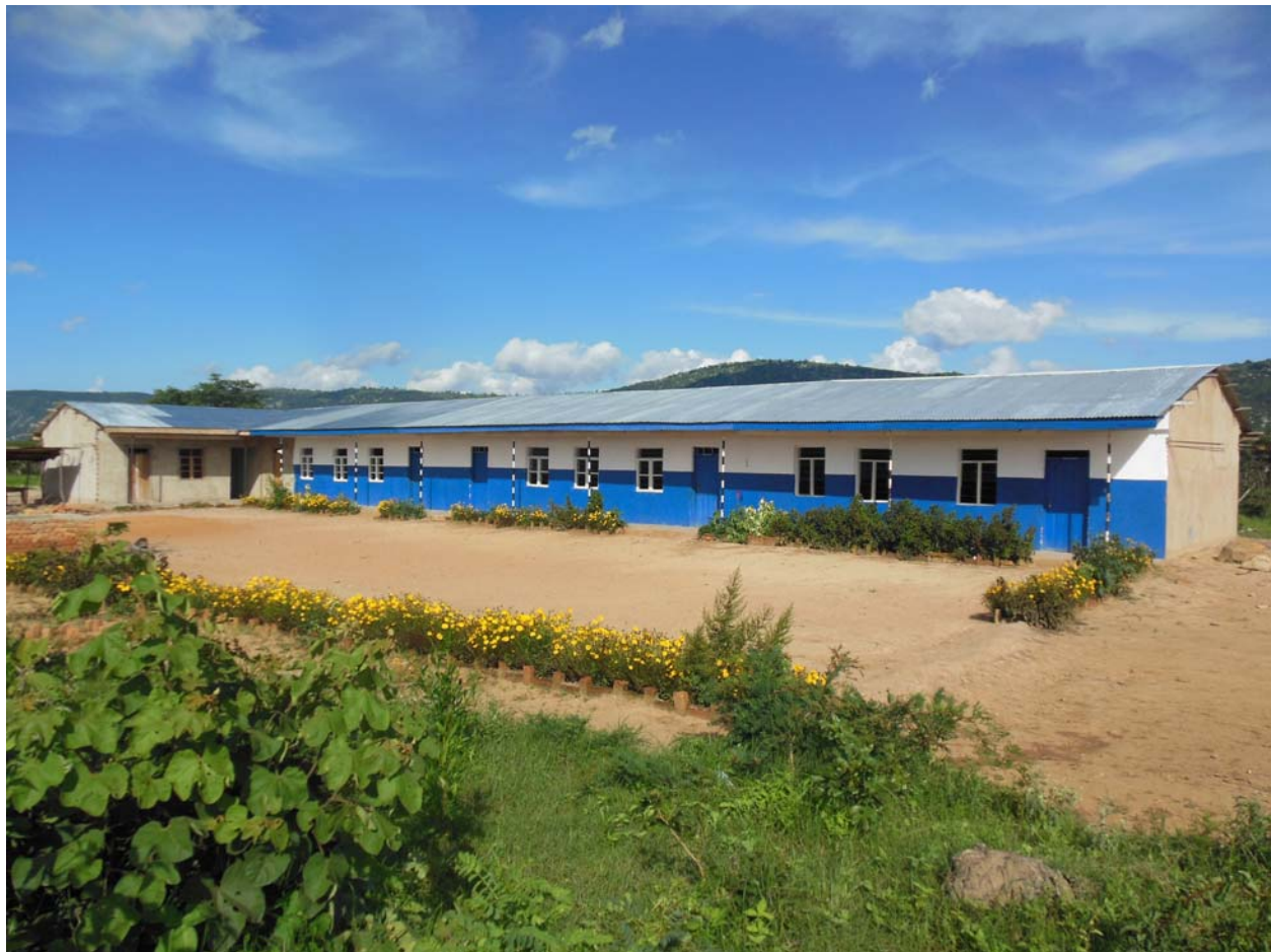
The Kibati Primary School with the new fourth classroom and second teachers' office (December, 2012).
