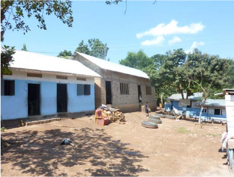
The new classrooms at Little Angels Primary School nearing completion.
