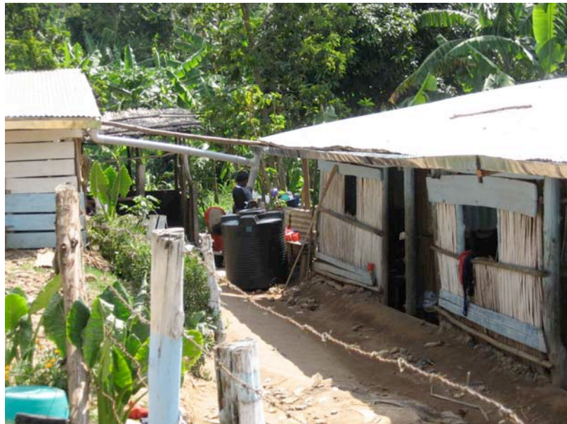
This shows some of the classrooms at Little Angels and the new rainwater catchment system.
